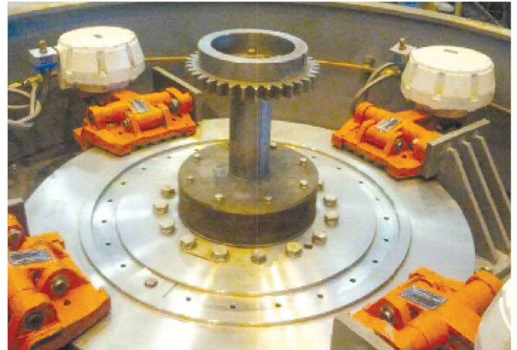
Kateel Pneumatic Disc Brakes mounted on 6000KW Pump Motor with a rated RPM of 1500 & max RPM of 1800 and a Braking torque of 30,000 N m used in Nuclear power plant.
