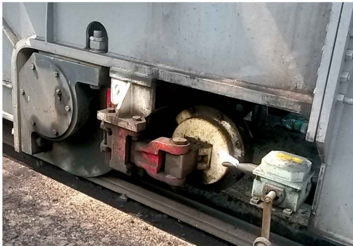
Hydraulic Disc Brakes mounted on Trippler Wheel in Port Conveyor
